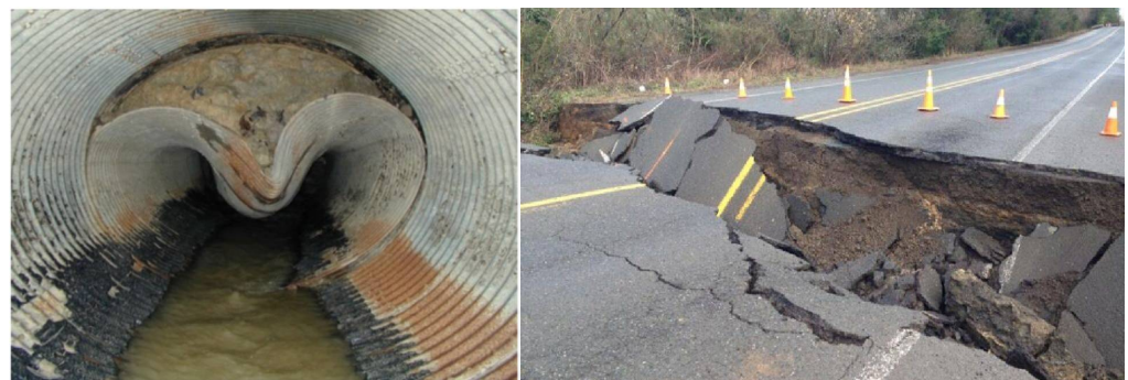
Figure 1. Left: culvert collapse on I-480 in Cleveland (USA) in 2001 [11]. Right: collapse of a culvert in Oregon (USA) in 2016 [12].
